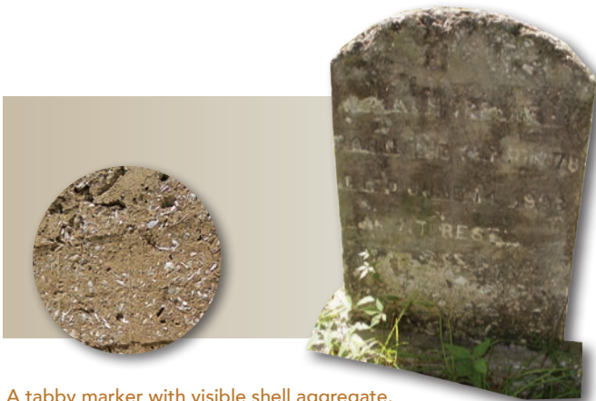
A tabby marker with visible shell aggregate.
